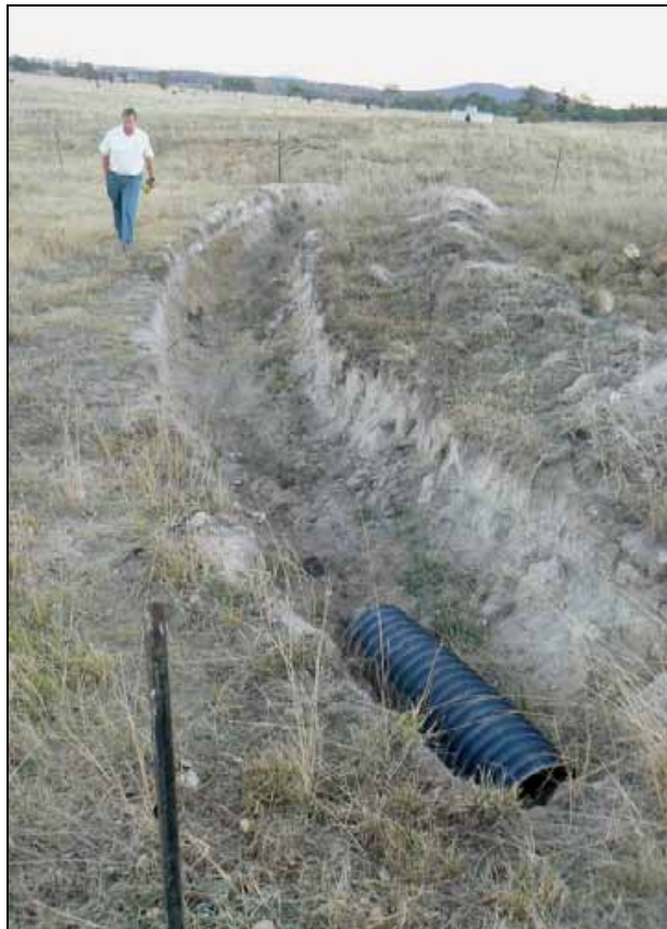
Fig. 2. An unfinished absorption trench. (From: Design and installation of water waste systems, Sydney Catchment Authority).
